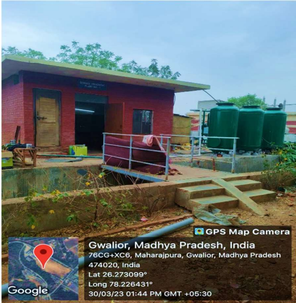
Sewage Treatment Plant
